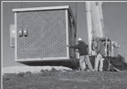
Housed Pump Systems
