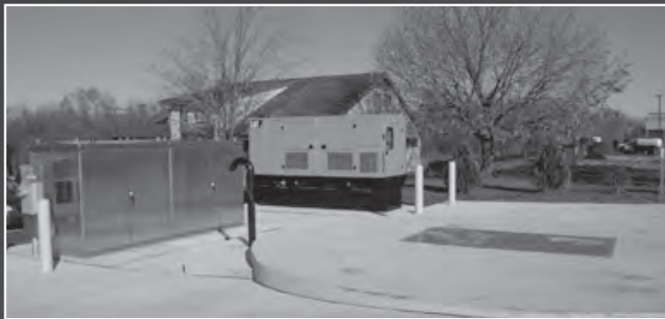
Lift Stations—New and Retro-fit Upgrades
